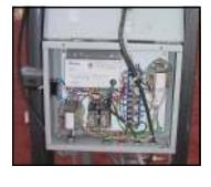
ELECTRONIC CONTROL IS USED TO KEEP THE TP CAN OIL/WATER AT BEST SEPARATION TEMPERATURE AND TO AUTO IGNITE THE PILOT ON THE INTEGRATED PROPANE BURNER
