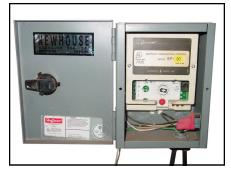
ELECTRONIC TEMPERATURE CONTROL IS USED TO KEEP THE TP CAN OIL/WATER AT BEST SEPARATION TEMPERATURE
