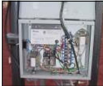
**ELECTRONIC CONTROL IS USED TO KEEP THE TP CAN OIL/WATER AT BEST SEPARATION TEMPERATURE AND TO AUTO IGNITE THE PILOT ON THE INTEGRATED PROPANE BURNER**
