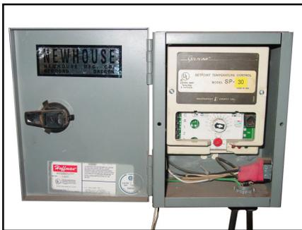
**ELECTRONIC TEMPERATURE CONTROL IS USED TO KEEP THE TP CAN OIL/WATER AT BEST SEPARATION TEMPERATURE**
